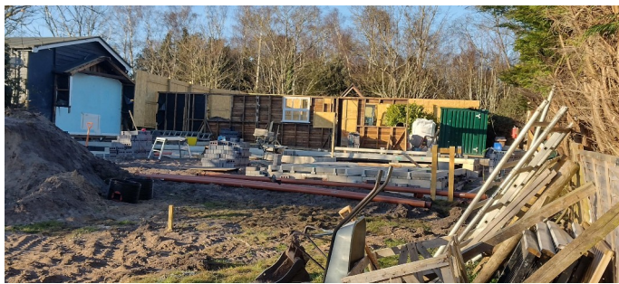
Caption:- Demolition and rebuilding works in The Uplands
