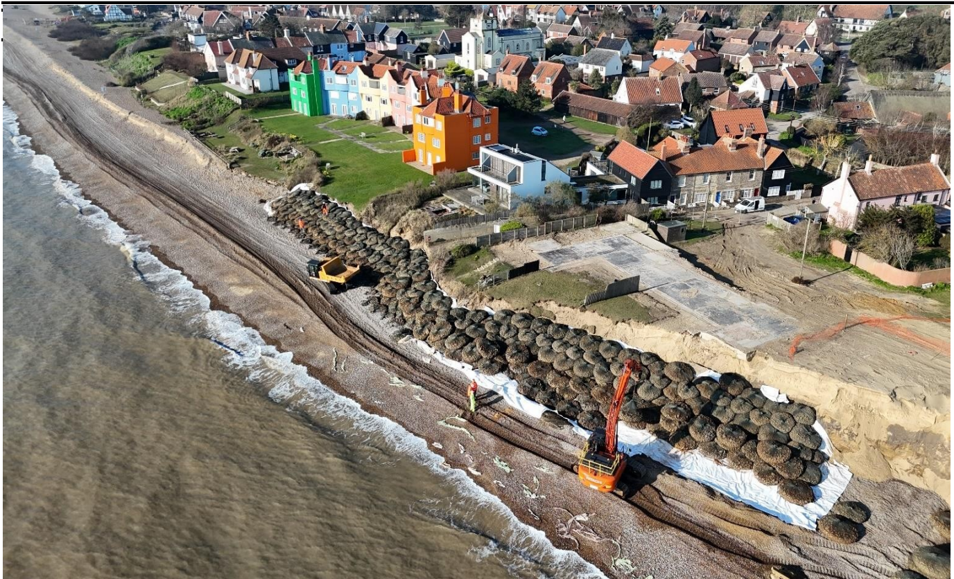
Defensive rock bags being installed at Thorpeness
