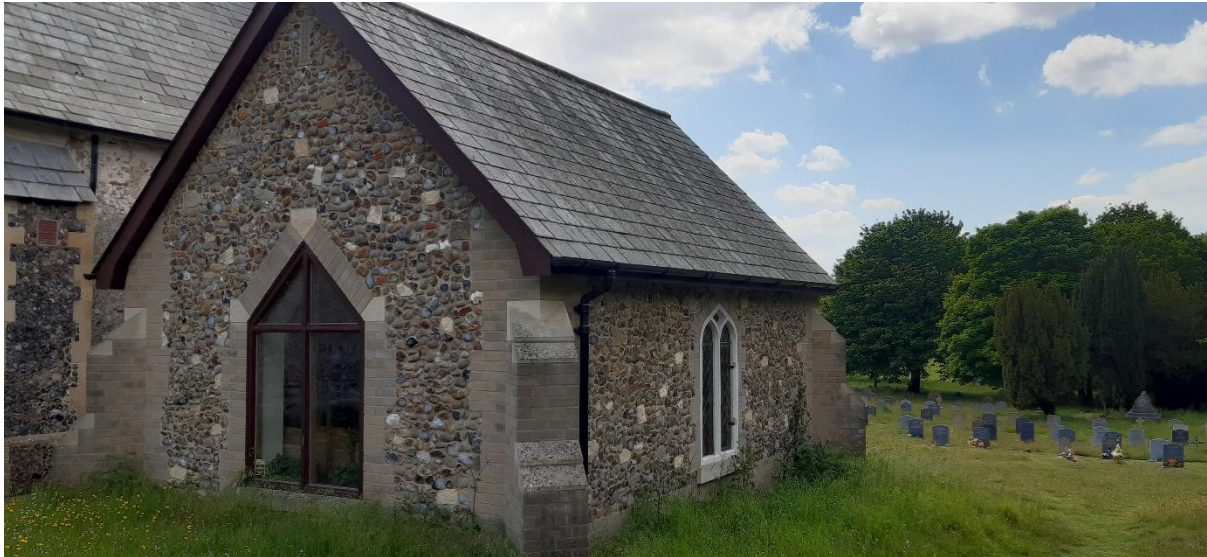
Figure 48: St Andrew's Church northern extension.
