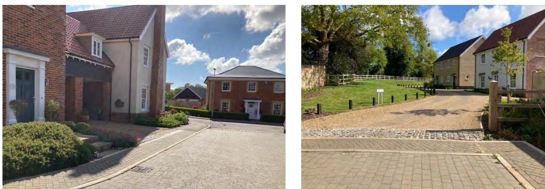
Figure 21: New development in Aldringham
