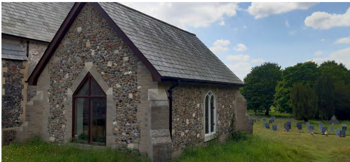
Figure 48: St Andrew's Church northern extension.
